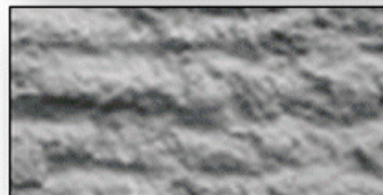
CSP 9 (heavy scarification)
