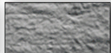
CSP 6 (medium scarification)
