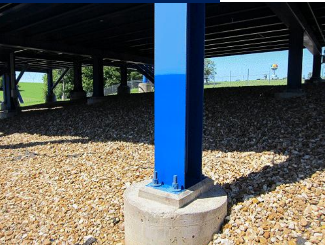
AFTER Application of Nano-Clear®
